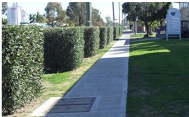
Footpath in Euroka Street alongside Council's Administration office
